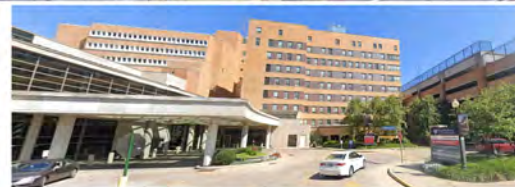
8 LGH EMERGENCY ROOM ENTRY
