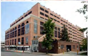
6 LGH PARKING GARAGE
