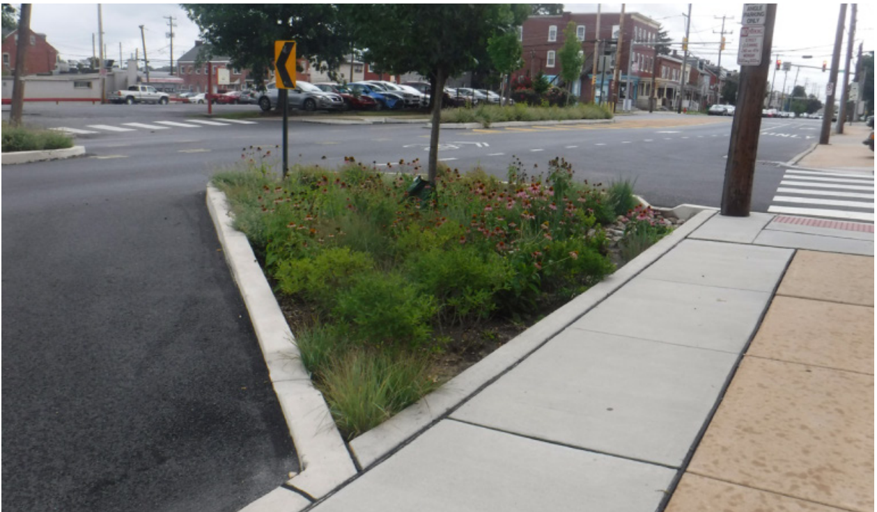
Figure 5.2-1. Typical Bioretention/Bioinfiltration System.
