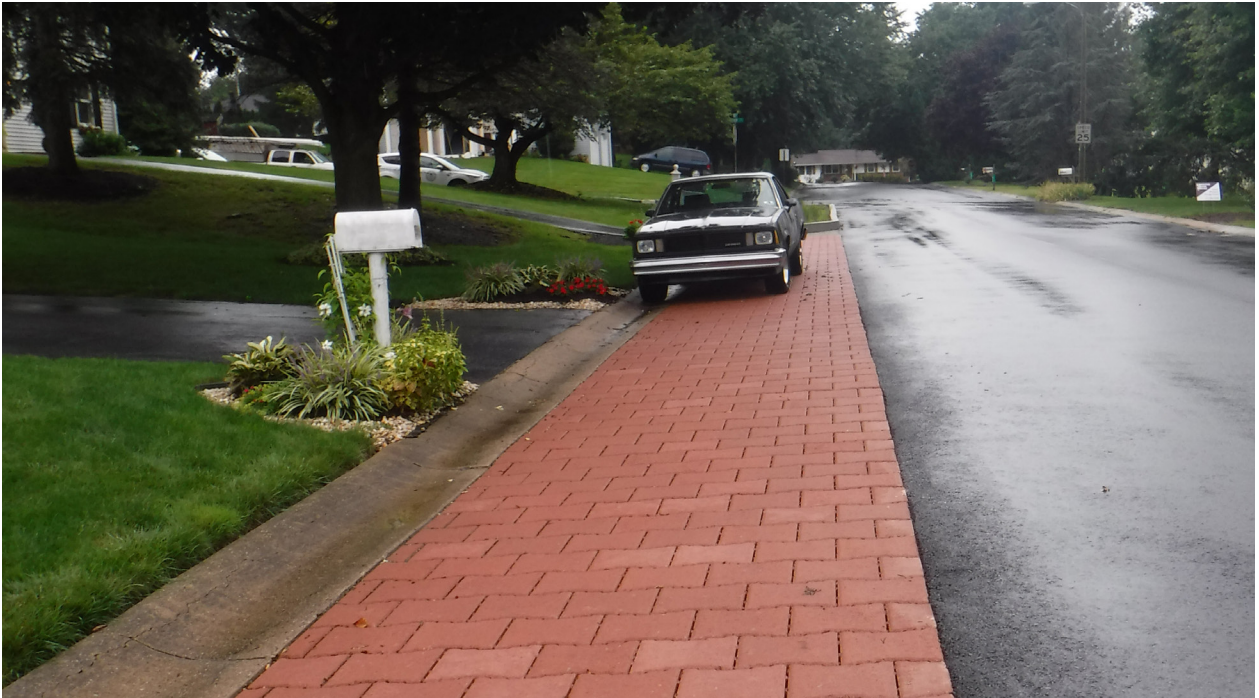
Figure 5.3-1. Typical Porous Pavement System
