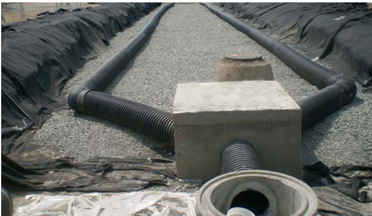
Figure 5.5-1. Typical Subsurface Infiltration and Detention System
