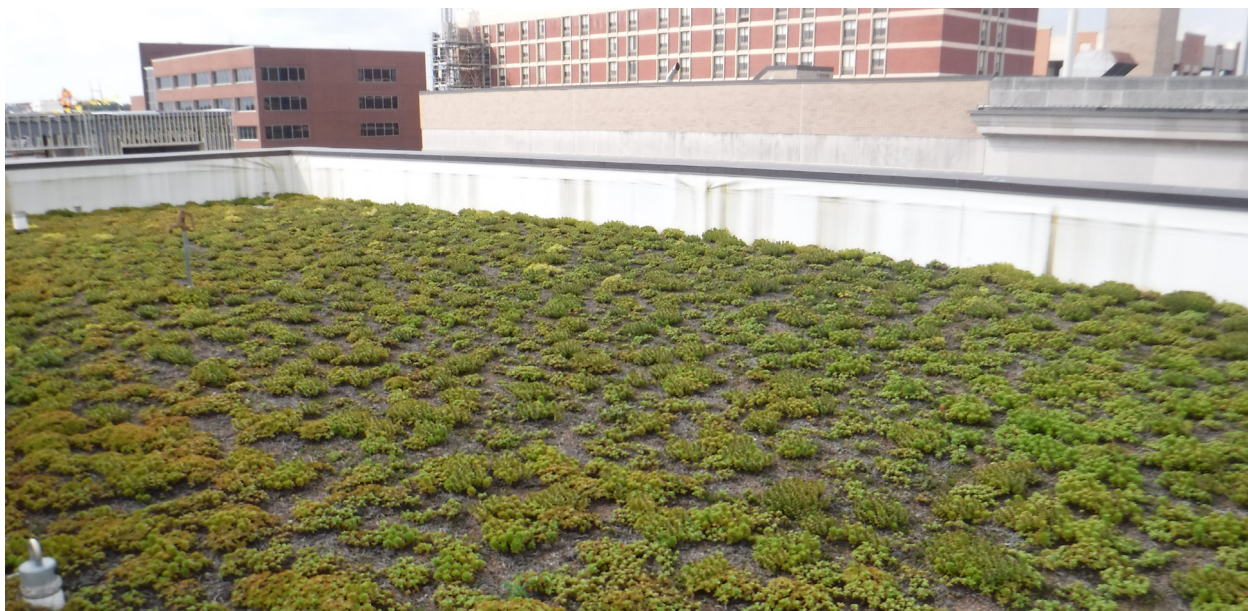
Figure 5.4-1. Typical Green Roof System
