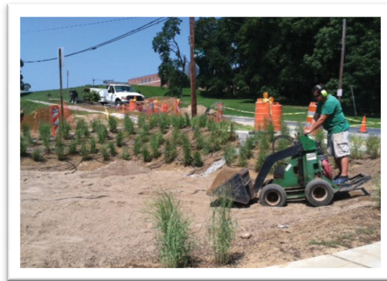
Bioretention and infiltration, Lancaster, PA Photo credit: Danielle Gallet, CNT
